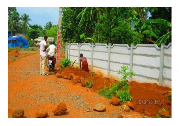
Earth work excavation for shifting water supply pipeline - 20.04.2011
